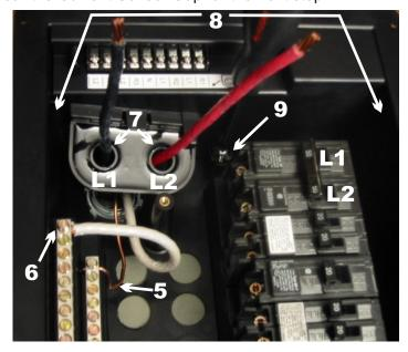
9) Secure Current Sensor/Barrier Wall Assembly to Housing using 8-32 X 7/16" screw provided.
